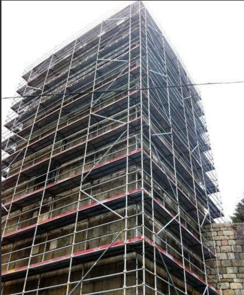
Gales, UK, HOS Construction
