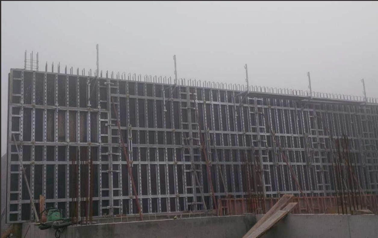
Industrial Building, Amarante, PT
